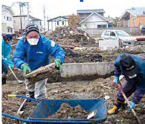
Employee Volunteers Clearing Debris and Mud
