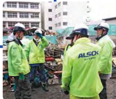
Employee Volunteers Clearing Debris and Mud at an Elementary School in Ishinomaki City, Miyagi Prefecture
